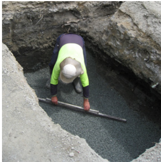
Left: Leveling the bedding
